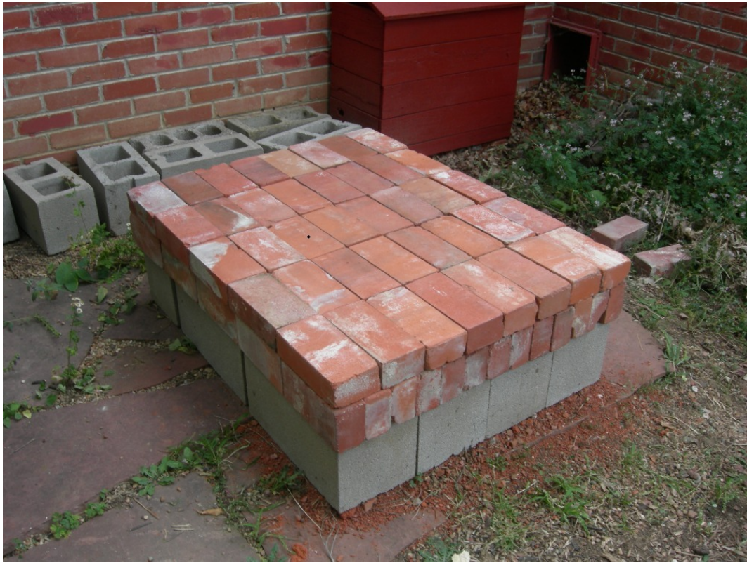
The second brick layer is 8 across, 5 deep, laid flat. This is the oven floor level.
