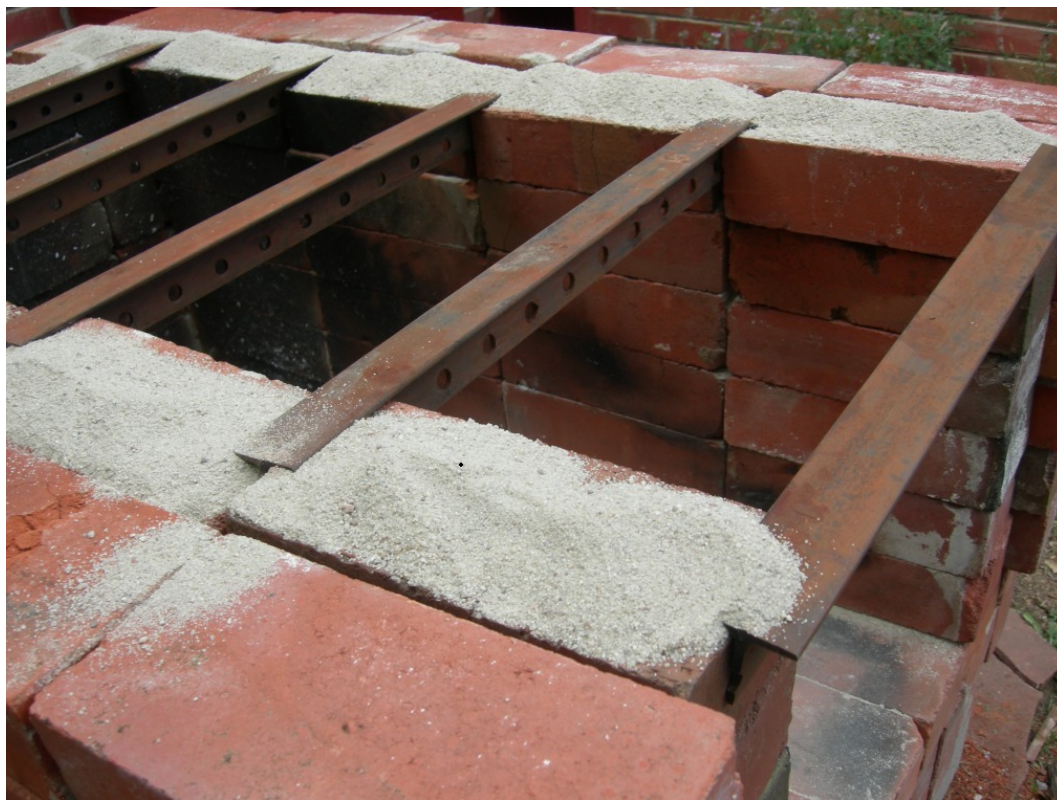
Showing the outer walls, T-iron roof supports, and sand or mortar used to fill between the T-irons. At this point we built a fire in it, just to make sure the bricks did not crack.
