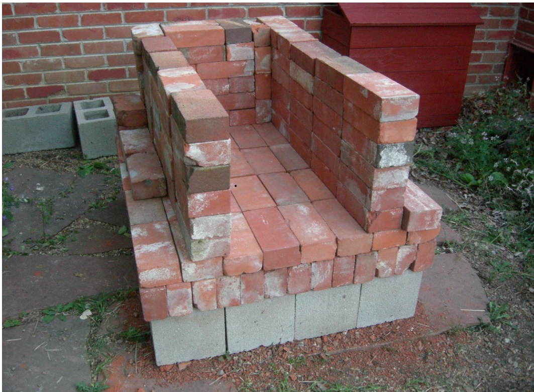
The inner walls of the fire box are 6 high, 5 deep, laid flat. The opening is 14 ½ inches. Note the slight overlap of the inner walls across the chink in the floor, to reduce air leaks.
